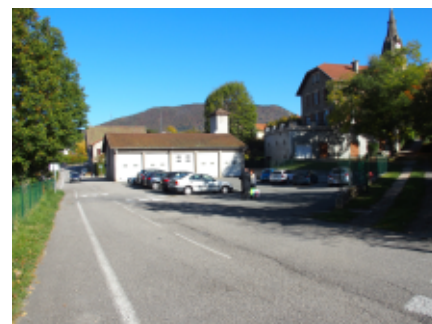
Large surface de parking imperméable
